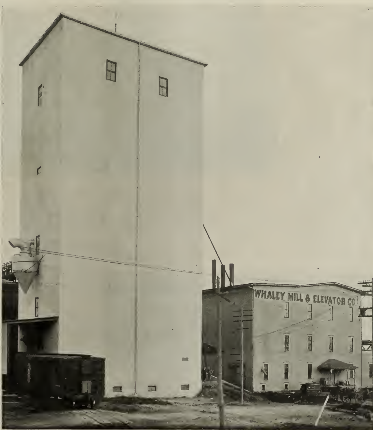
NEW ELEVATOR OF THE WHALEY MILL & ELEVATOR COMPANY, GAINESVILLE, TEXAS Designed and Constructed by the Macdonald Engineering Company, Chicago, Ill.
